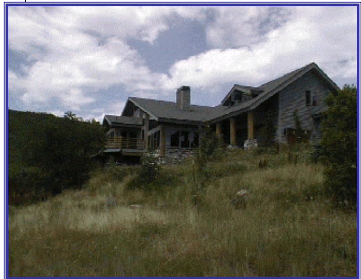
Landscape to retain harmony and preserve the original character.
